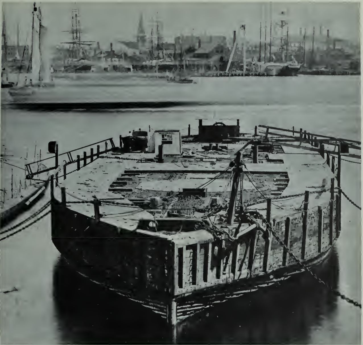
U.S. Monitor Miantonomoh lying at Boston in 1874—Her armor, turrets and other fittings have been removed and she is in reality only a hulk. At the same time construction of the second monitor to be named USS Miantonomoh was beginning.
